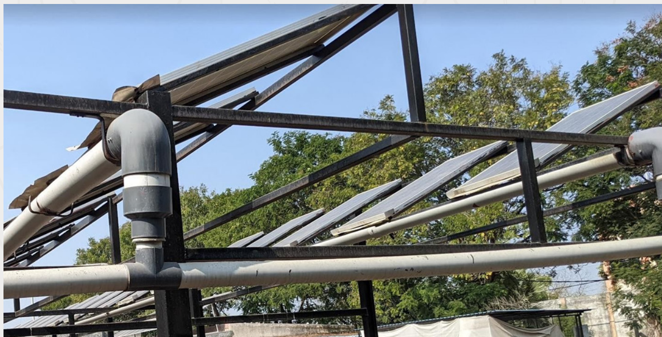
Figure 72. Installed pipe system to collect cleaning water (Credit: JAU)
