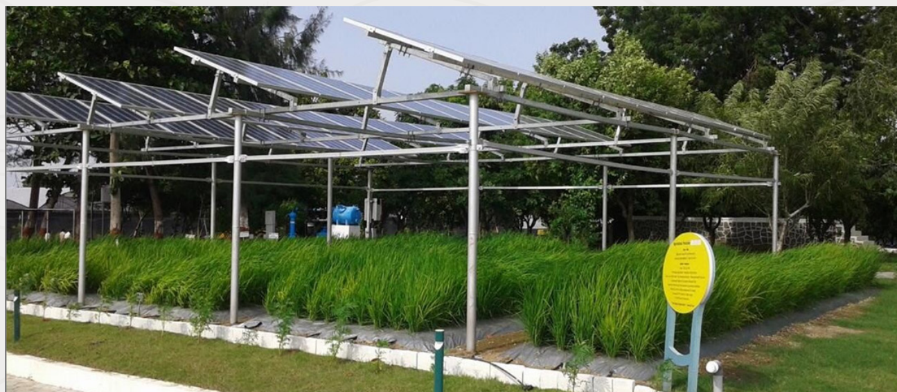
Figure 38. 9.6 kW Agrivoltaics system with rice (Credit: Jain Irrigation)
